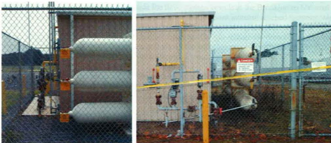
A View of the High Pressure Natural Gas Storage Vessels with the Failed Relief System Before (left) and Aft
